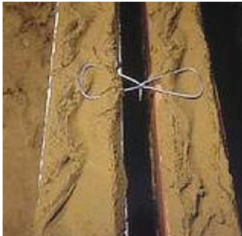
Fig2—Wall tie installation
