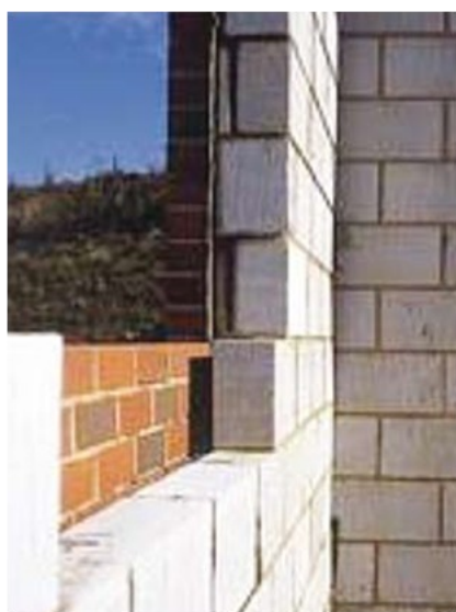
Modern cavity walls under construction.
