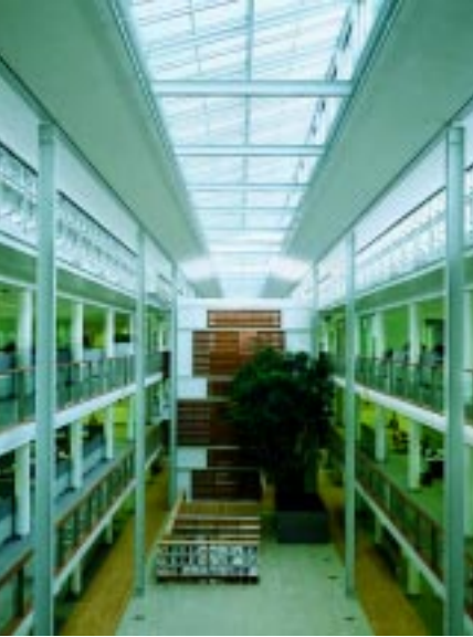
Figure 3 The central atrium at Powergen's Head Office allows for natural ventilation via motorised openings at high level
