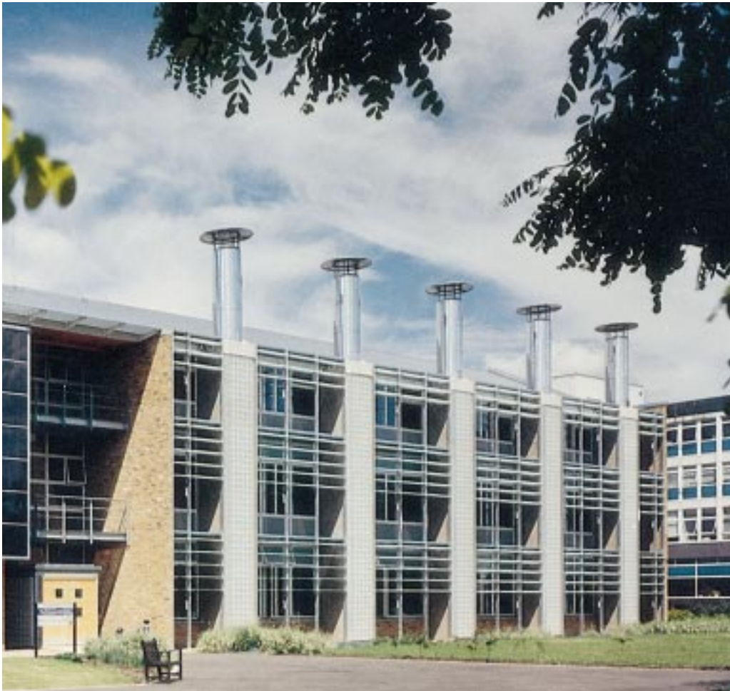
Figure 1 BRE Environmental Building – showing ventilation stacks and external solar shading
